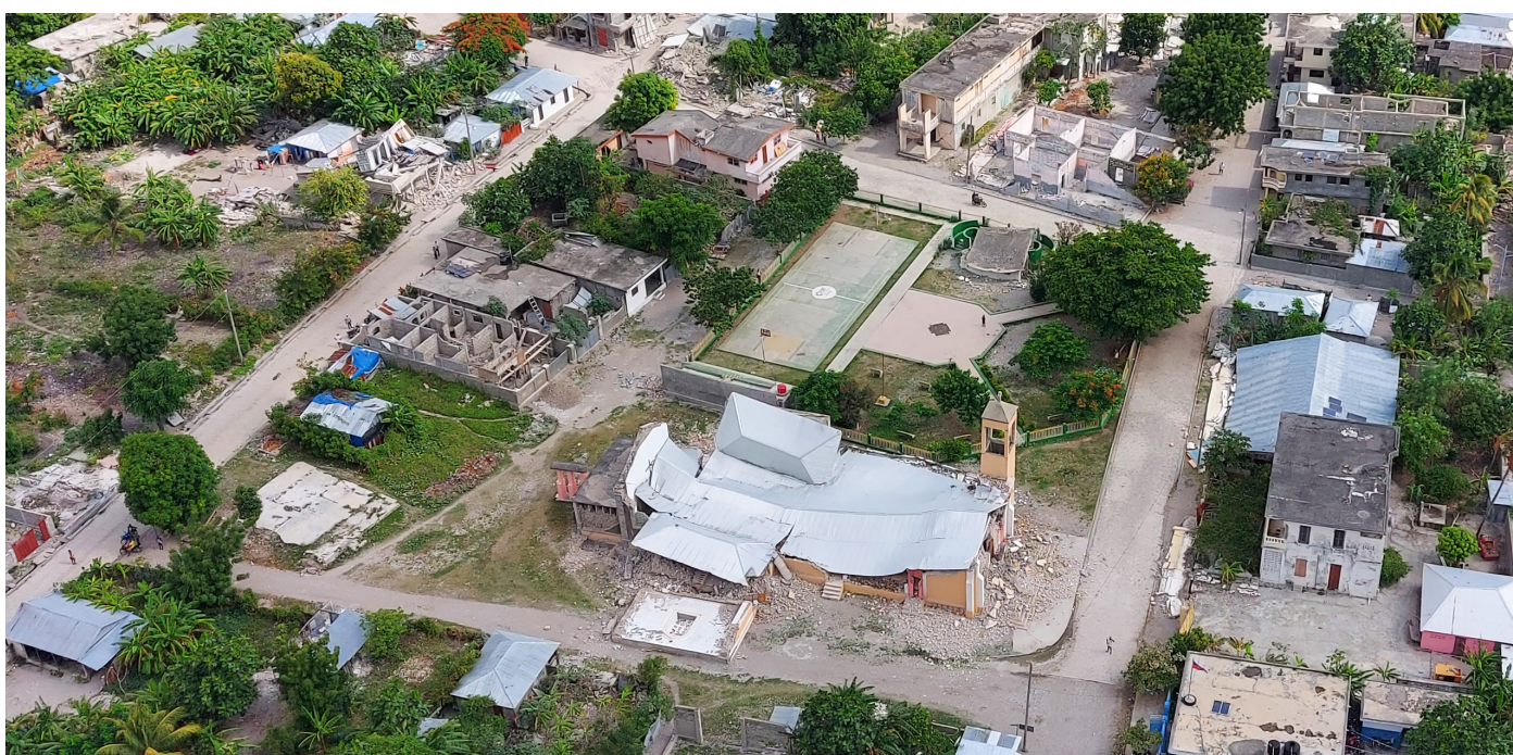
Collapsed church in Les Cayes © IOM 2021
